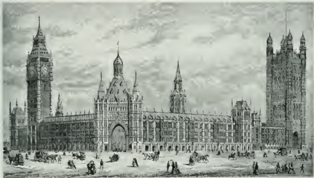
VIEW OF BUILDINGS DESIGNED BY HARRY TO ENCLOSE NEW PALACE YARD ( p. 536).
